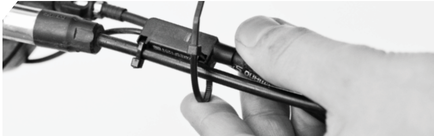
Figure 13: Installing the Switch Junction Box
